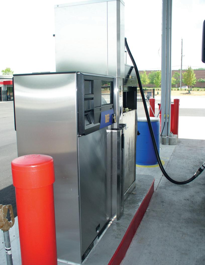
Wayne DEF dispensers use a patent-pending heated hose and nozzle enclosure with automatic door operation for easy access.
